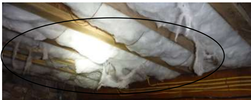
Figure 12 Insulation, wire hangers and metal in crawl (plumbing, strapping, etc.) was rusted; high humidity & seepage in crawl space. Recommend a wet crawl space contractor evaluate crawl and advise on dehumidification, ventilation and water management system.
