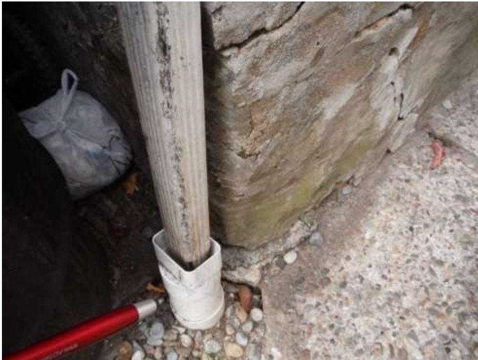
Figure 4 Foundation cracks corner in rear left side by bowed wall.
