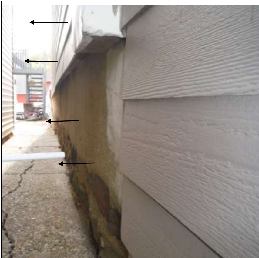
Figure 3 Bowed wall and foundation; left side building. Recommend a structural mason evaluate foundation and advise on repair, repointing, etc. Have a siding contractor or qualified building contractor evaluate bowed wall, loose siding and advise. Recommend a structural engineer (PE) evaluate structure and advise on any structural repairs.
