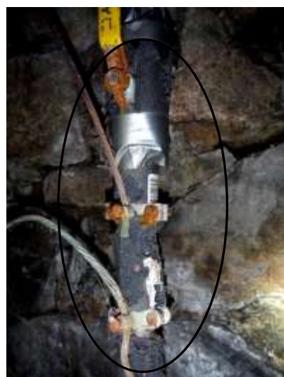
Figure 18 Example of corrosion on water meter, piping, fittings, ball valve(s), black gas piping, etc. Crawl was wet/seepage/high moisture and poor ventilation; conducive to rust/corrosion, potential structural structure/water damage and attracting wood destroying insects. Insulation in ceiling was sagging & moist; have evaluated for dehumidification and ventilation (poor). Pipe insulation was chewed; mice or rodents.
