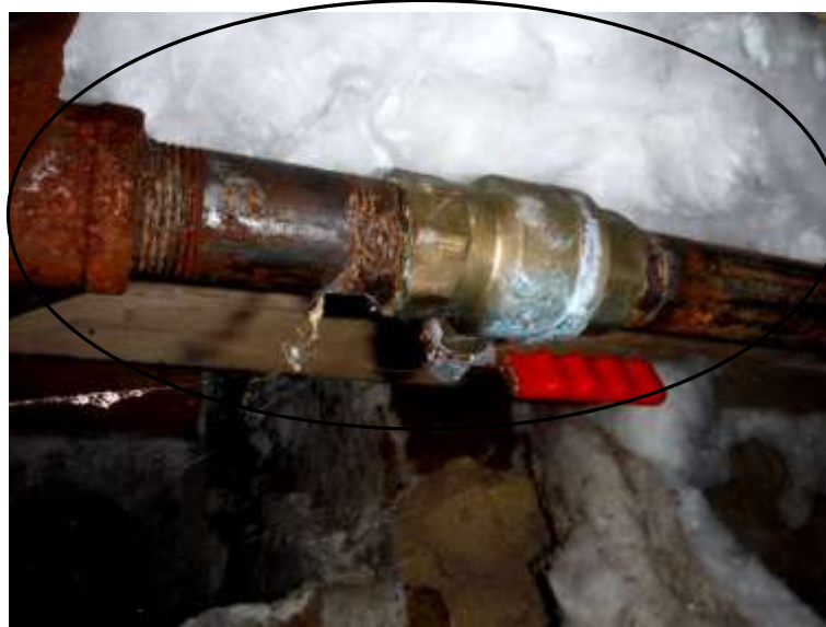
Figure 18 Example of corrosion on water meter, piping, fittings, ball valve(s), black gas piping, etc. Crawl was wet/seepage/high moisture and poor ventilation; conducive to rust/corrosion, potential structural structure/water damage and attracting wood destroying insects. Insulation in ceiling was sagging & moist; have evaluated for dehumidification and ventilation (poor). Pipe insulation was chewed; mice or rodents.
