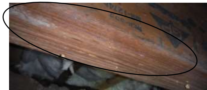
Figure 14 Example of gray film and darkening on joists and framing in crawl; possible mold.
