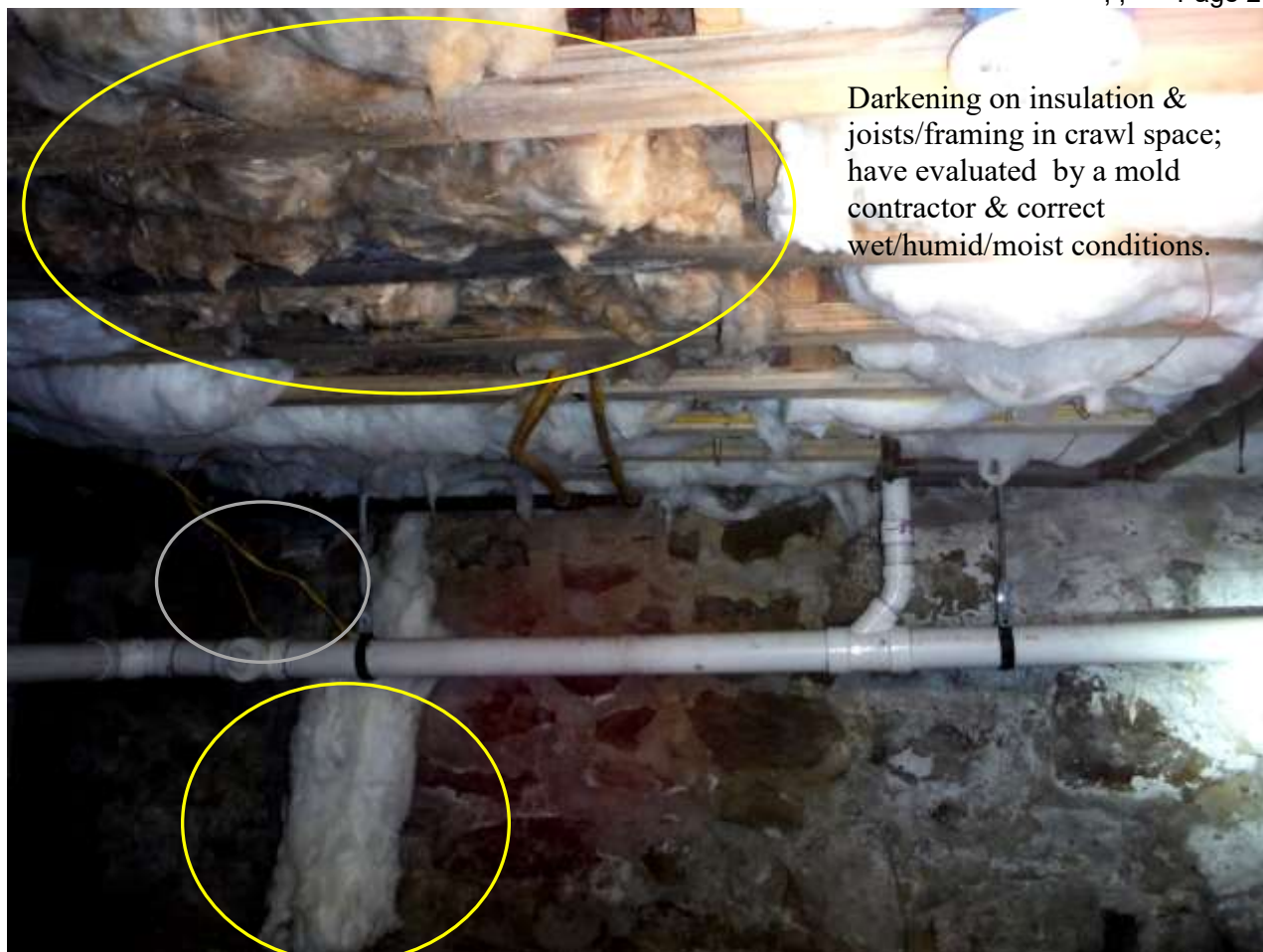
Figure 13 Loose/hanging insulation, sagging/moist insulation. Darkening on fiberglass insulation; possible mold/mildew. There were loose electrical wires; have secured where needed. Crawl was wet/seepage and insulation, plumbing, metal (insulation hangers, strapping, etc.) was corroded or rusted. See plumbing section; corrosion on plumbing and water meter.
