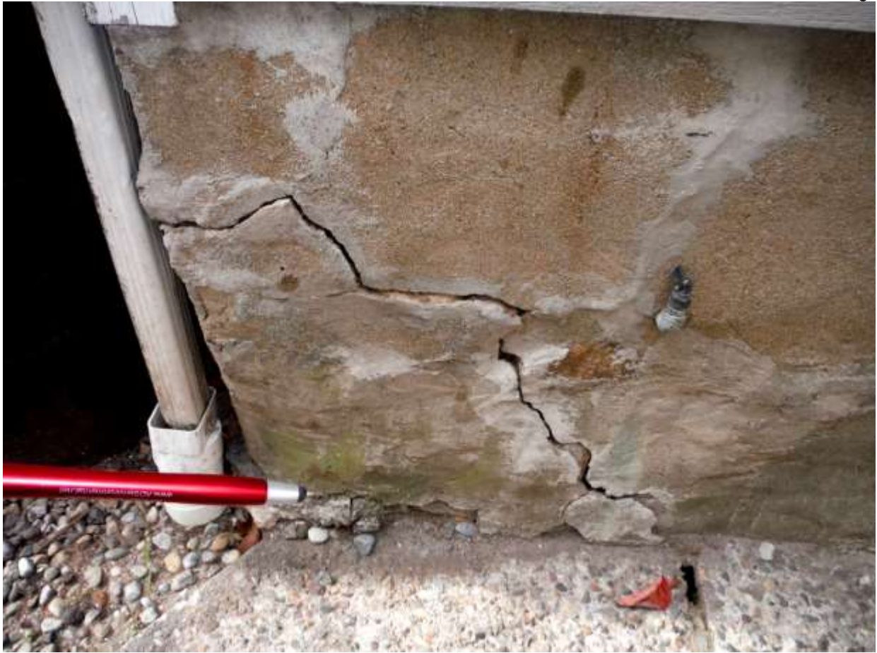
Figure 4 Foundation cracks corner in rear left side by bowed wall.
