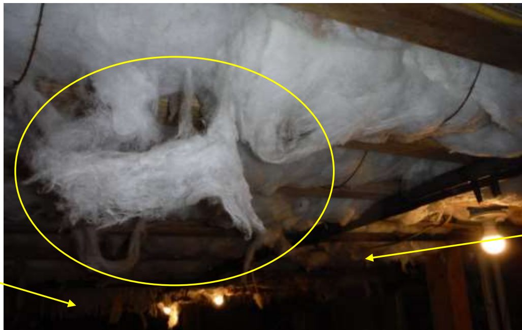
Figure 12 Insulation, wire hangers and metal in crawl (plumbing, strapping, etc.) was rusted; high humidity & seepage in crawl space. Recommend a wet crawl space contractor evaluate crawl and advise on dehumidification, ventilation and water management system.
