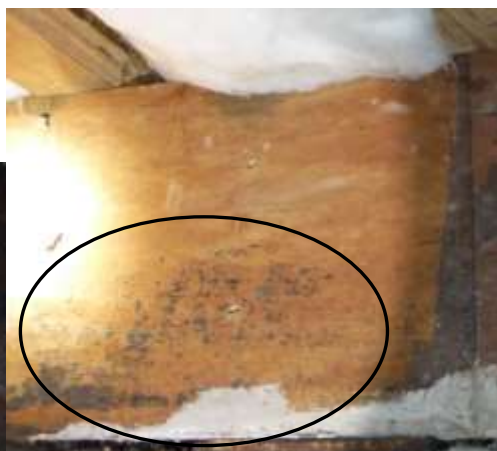
Figure 14 Example of gray film and darkening on joists and framing in crawl; possible mold.
