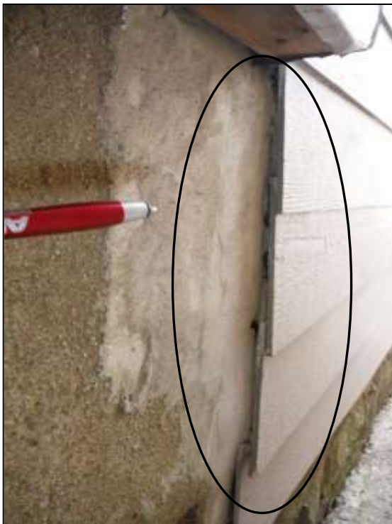
Figure 3 Bowed wall and foundation; left side building. Recommend a structural mason evaluate foundation and advise on repair, repointing, etc. Have a siding contractor or qualified building contractor evaluate bowed wall, loose siding and advise. Recommend a structural engineer (PE) evaluate structure and advise on any structural repairs.
